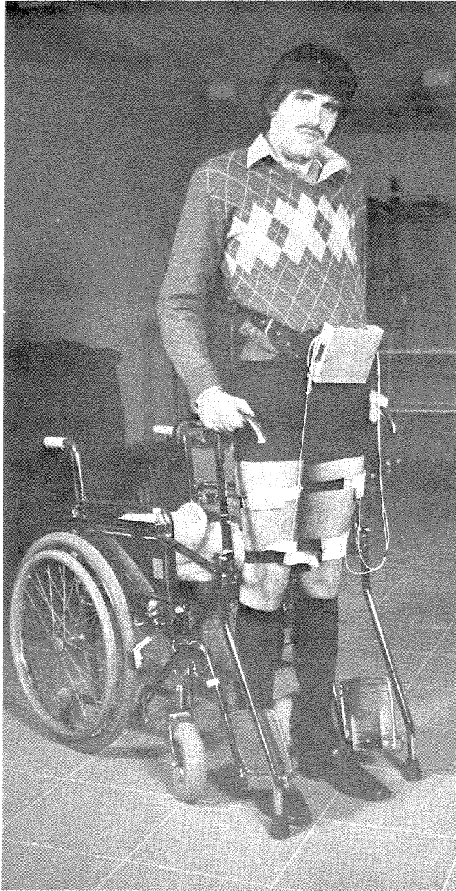
FIGURE 1 Standing by means of FES and the wheelchair-attached supporting frame.
